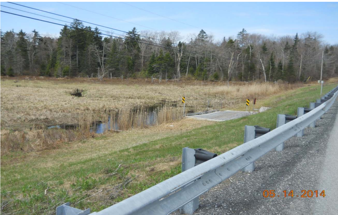
Looking Southwest at Snowmobile Bridge
