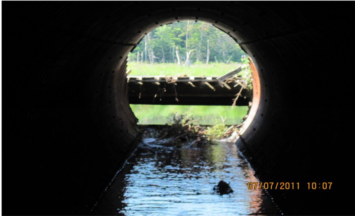
Interior of Pipe Looking at Snowmobile Bridge
