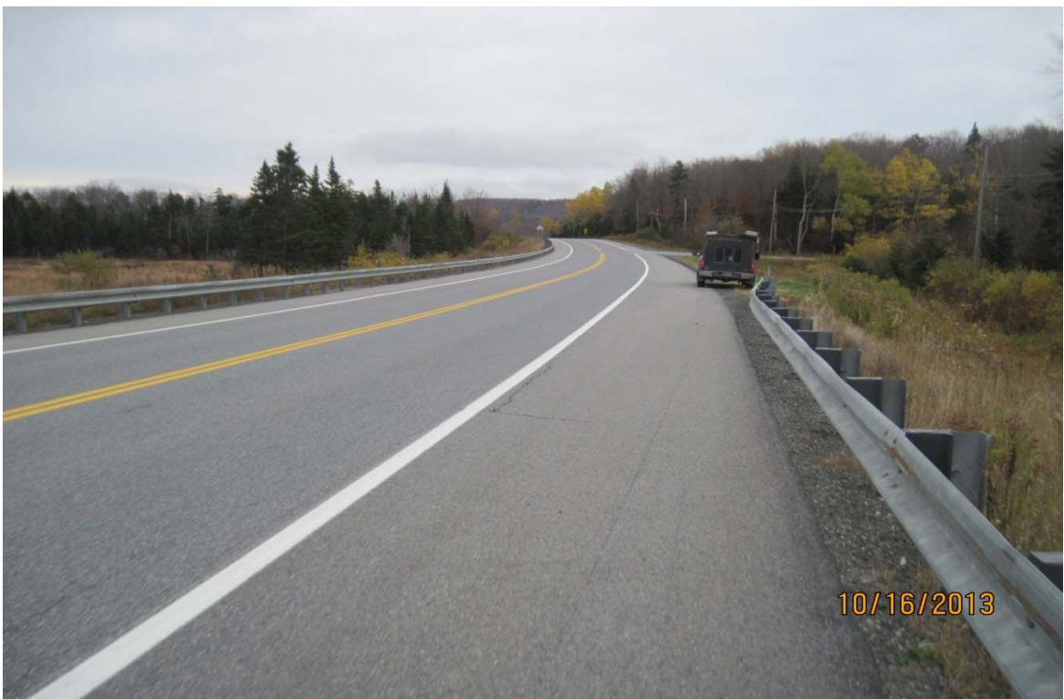
VT Route 9, Looking East
